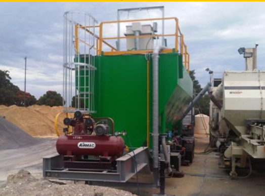
Silo and hopper in working position feeding mixture
