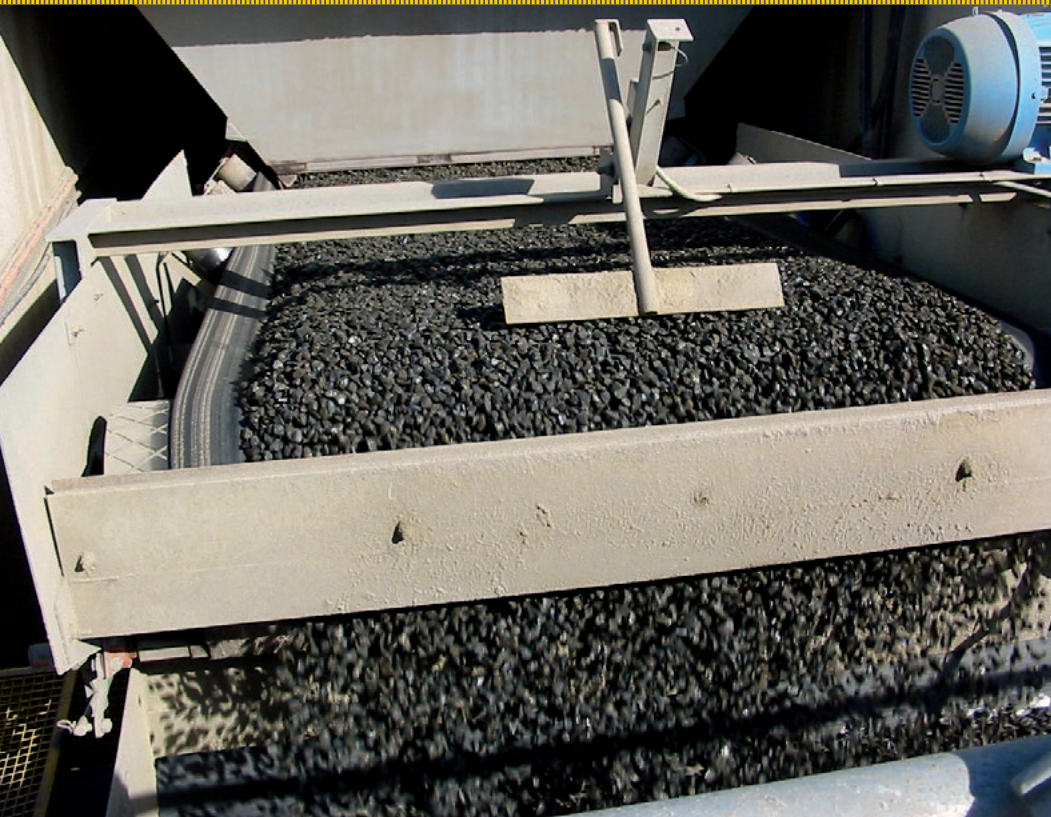
20mm aggregate feeding onto discharge conveyor
