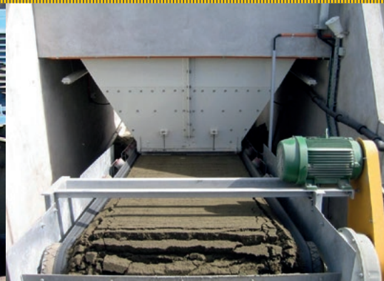
Sand feeding onto discharge conveyor
